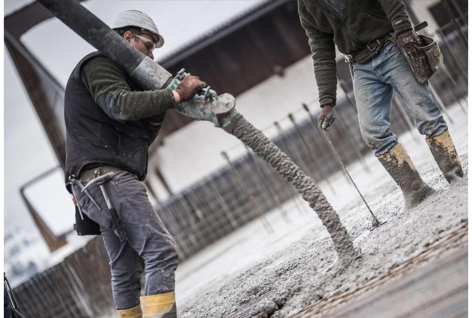
A photograph showing two construction workers on a site. One worker in the foreground is wearing a grey hard hat, safety glasses, a dark jacket, and grey pants, and is using a long, flexible concrete pump hose. Another worker in the background is wearing blue jeans and yellow boots, and is using a tool to guide the concrete. The background shows a building under construction with rebar structures.
